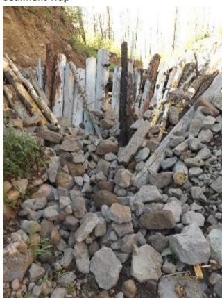
Sediment trap structures are placed often in highly active channels that are moving large sediment. Keeping large amounts of sediment out of the main Santa Clara Creek benefiting aquatic ecology.
