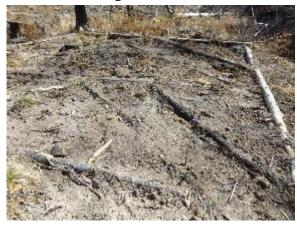
In areas where dirt is needed to build berm structures, a basin can be dug in a location where there is excess runoff. Basins collect and allow water to seep gradually into the subsurface instead of remaining on the surface where erosion can occur. There are many different types of water harvesting designs, the photo to the left, is a delta structure designed to encourage alluvial deposition.
