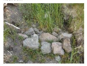
Rocks are positioned in various ways, used not only to prevent erosion but also to aggrade the streambed creating viable habitat for plant life. Note; healthy vegetation thriving upslope of rock dam structure in photo to the left. Rock dams are commonly used in tributary headwaters within swallow eroded channels. Rock dams are often of varying sized depending upon channel width.
