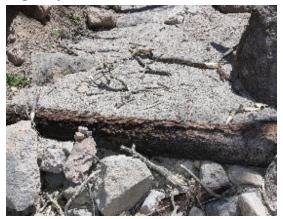
Log drop structure act similarly to rock dams, the log acts as a footer that is anchored into the banks of the incised channel. Rocks and dirt are manually placed upstream of the log and sometimes grass transplants are installed into the structure. All of these materials collaborate to collect sediment behind the log structure. The sediment collected contains rich organic materials such as seeds, animal manure, detritus material and other nutrients needed for healthy plant growth.
