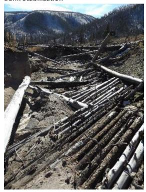
Bank stabilization structures are often used to protect one stream bank while increasing lateral erosion on the opposite bank. These structures are used to stabilize very specific stream banks that are fragile or in danger of being eroded into other channels, which is the case in the photo to the left. Logs can be positioned to encourage plant growth and slow down water along eroded banks.
