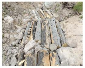
Logs placed parallel, into the channel and are anchored in with rocks and dirt, protecting streambed from eroding. Log mattresses are versatile erosion control structures which are easy to construct and have great value to the recovering ecosystem both in the short and long term. In the short-term, these structures collect sediment and raise the streambed. In the long-term, log mattresses will decompose providing organic material encouraging plant growth.
