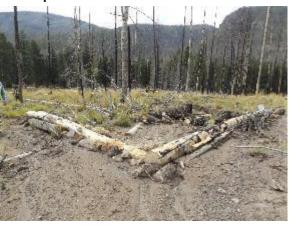
Flow splitters work similarly to diversions keeping flow out of a main incised channel and can encourage sheet flow. These designs are most effective in wide valley bottoms where flow has space to spread and dissipate. (Refer to Log Diversion description previously mentioned.)
