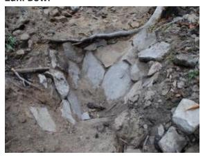
Constructed at the base of a head-cut, Zuni bowls (originally used by Zuni Pueblo) armor the substrate within the channel, preventing scouring action by water over the long term. The bowl shape acts as an energy dissipater as water flows into the structure, protecting the potentially erosive substrate. The bottom of the bowl also acts as a water harvesting feature which will maintain moisture for longer periods.
