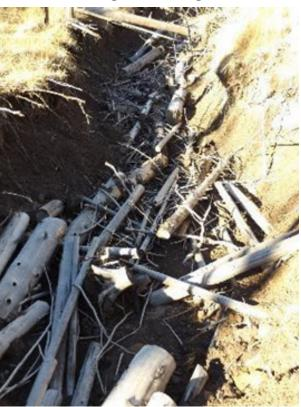
In deep incised channels that are difficult or dangerous to work in, and in areas where there is an abundance of deadfall directional felling and bucking can be implemented to safely and quickly treat an erosive system. Ideally over long periods of time these logs will decompose adding organic material back into the system. Seeds can sometimes germinate within the various niches of these logs.
