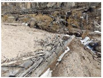
The main function of a meander inducing structure is to decrease vertical erosion and encouraging lateral erosion (which is a good thing) with in a channel. Meander inducing structures increase the flow length which allows the water to slow and have more time to deposit sediment.
