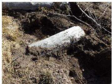
Head cuts are very problematic and can cause excessive erosion that continue to erode up drainage losing large amounts of soil. To prevent further head cutting, logs and rocks can be placed upstream to keep soil in place and stop a head cut from migrating further.
