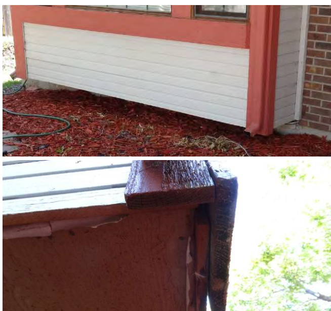
Figure 28: The "bump out" design feature at the front of the Rossmere Street home would be been vulnerable, if the wood mulch had been ignited by the observed ember exposure. Given the low earth-to-wood clearance, flame spread to the bump out would have provided a flame contact exposure to the combustible underside feature. Source: IBHS.
