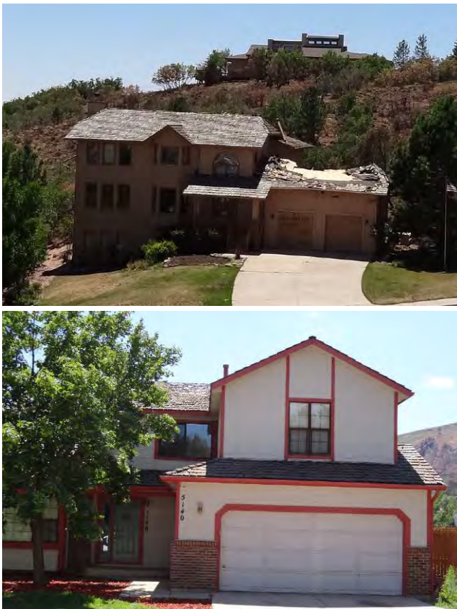
Figure 25: Homes on Rossmere Street (upper) and Champagne Drive (lower), each had wood shake roof coverings that were ignited by wind-blown embers. Source: IBHS.
