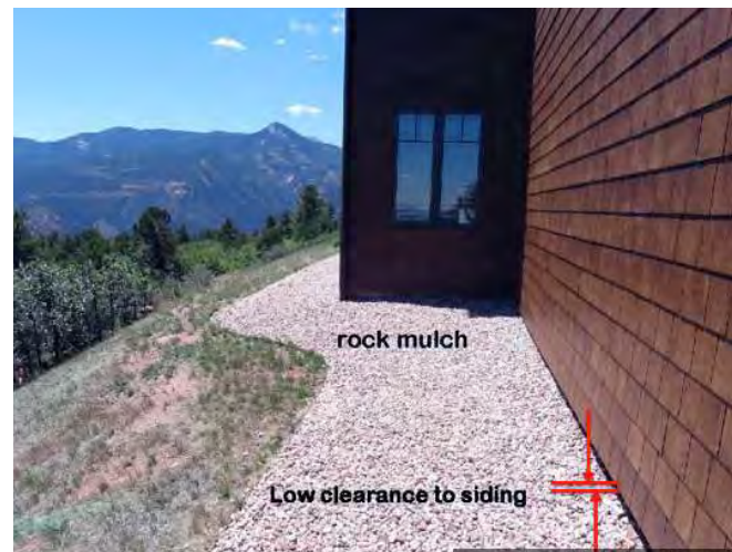
Figure 22: The back side of the home on Outer Vista Point Road. Noncombustible rock mulch and fiber-cement shingle siding products were used. The low clearance may allow for the underlying wood-based sheathing product to be vulnerable to ember accumulation at the base of the wall. Source: IBHS.
