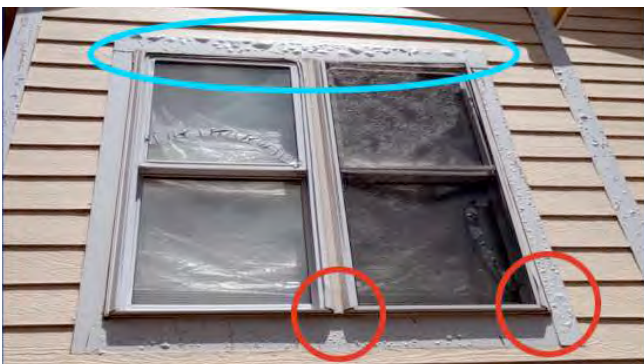
Figure 13: Radiant heat from the burning home, which was destroyed and was located 20 feet from this damaged home, was sufficient to cause paint on the wood trim to bubble (circled blue) and thinner components on the vinyl window frame to deform (circled red). Source: IBHS.
