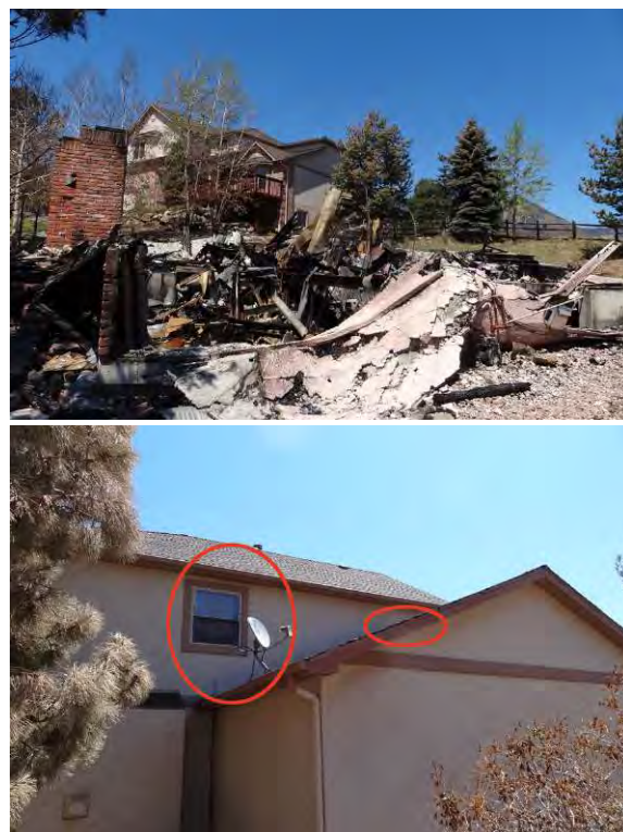
Figure 18: A composite figure of two damaged homes on the west side of Courtney Dr. The up-slope home is above and the down-slope home below. The charred combustible siding in the up-slope home is not visible in this figure. The damaged components in the down-slope home are circled. Source: IBHS.
