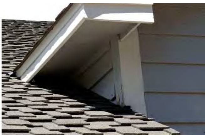
Figure 23: The roof-to-siding return on this complex roof consists of a composite wood (hardboard) siding product and a Class A fire-rated asphalt composition shingle roof covering. Even without vegetative debris at the roof-to-wall intersection, an accumulation of embers could result in ignition of the wood-based siding. Source: IBHS.
